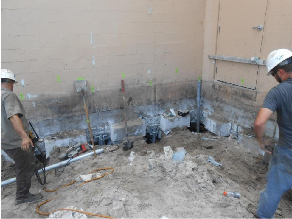
**Photo 5, Installation of underpins and foundation brackets along existing building**
