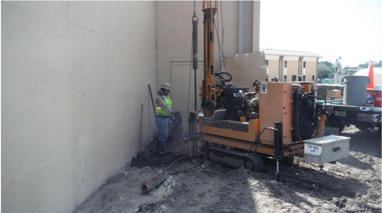
Photo 1, MEG completing a difficult access SPT boring adjacent to existing building
