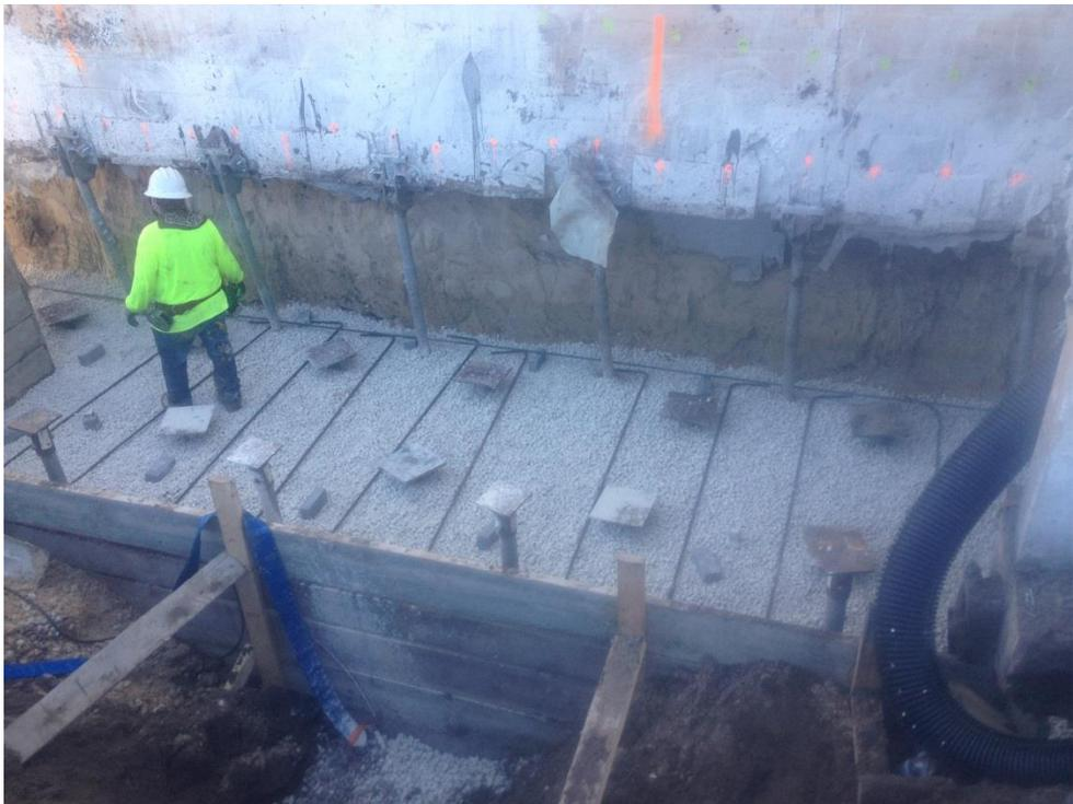
**Photo 6, Construction of pile cap for micropiles adjacent to existing building**
